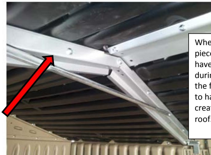
When the front roof connector metal piece (GG) and the front roof panels have not been properly aligned during assembly, this may be because the front roof connector metal piece to hang lower than it is supposed to, creating interference with the back roof.
